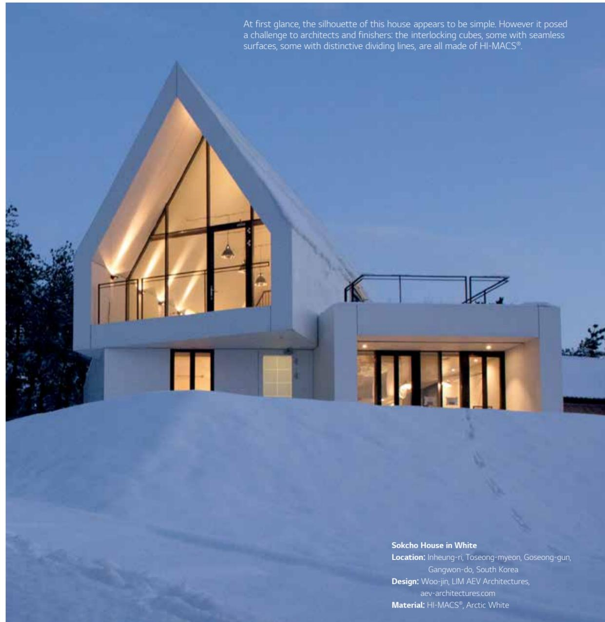
At first glance, the silhouette of this house appears to be simple. However it posed a challenge to architects and finishers: the interlocking cubes, some with seamless surfaces, some with distinctive dividing lines, are all made of HI-MACS®.
